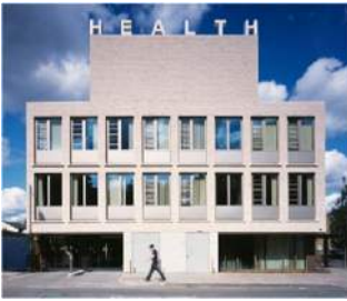
Akerman Road Health Centre, London, UK Client Lambeth, Southwark, Lewisham NHS Tranche 2 Lift Schemes Services Building services and fire engineering and sustainable design Architect Henley Halebrown Rorrison
