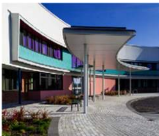
Grangewood Acute Mental Health, Belfast, Northern Ireland, UK Client Western Health and Social Care Services Building services engineering and sustainable design Architect Avanti Architects and Kennedy Fitzgerald Architects
