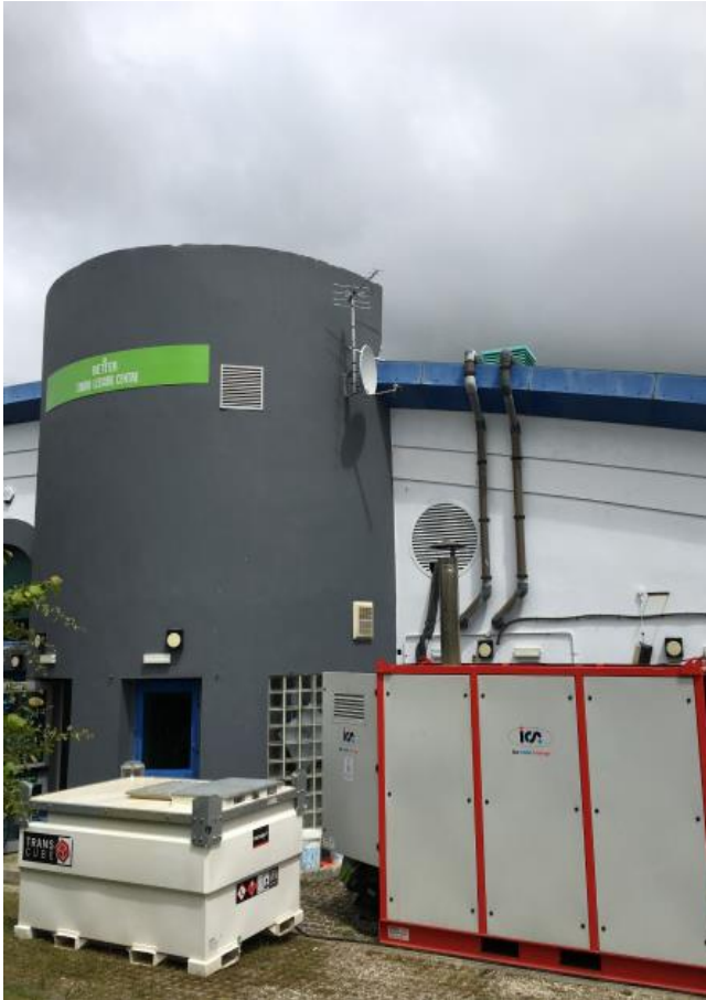
Boiler supplying essential temporary heating to a leisure centre
