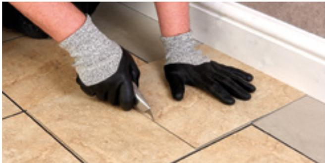
Figure 6 Measuring using an overlapping tile
