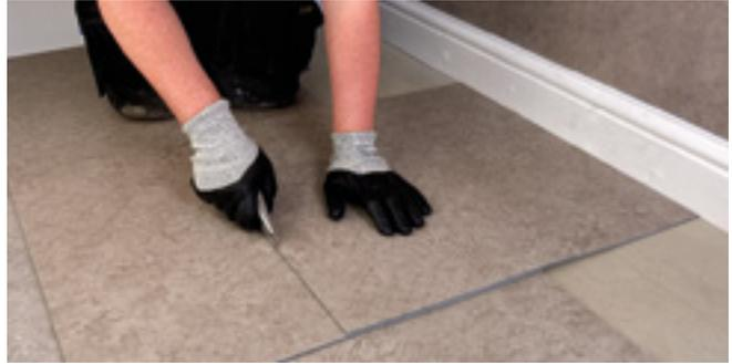
Figure 8 Measuring using an overlapping tile
