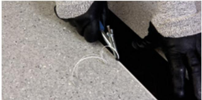
Figure 1 Grooving the seam
