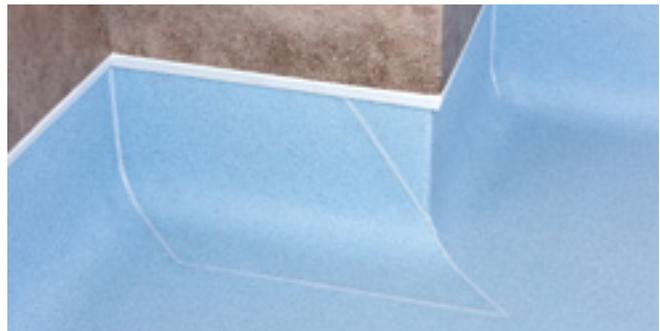
Figure 11 External corners 'wrap around method'
