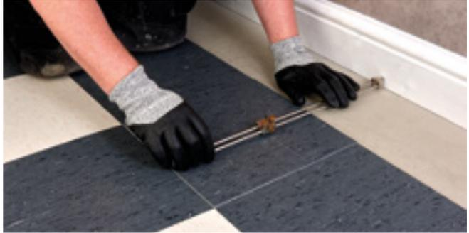
Figure 6 Measuring a tile using a scriber
