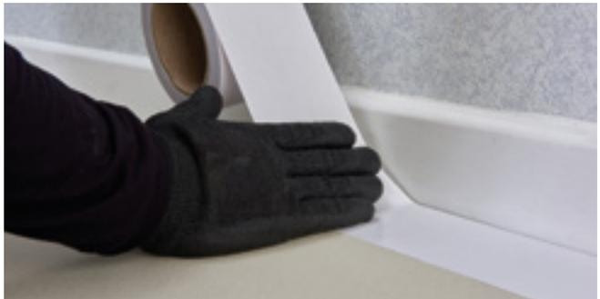
Figure 36 Use double sided QuickLay tape
