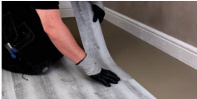
Figure 1 Setting planks out
