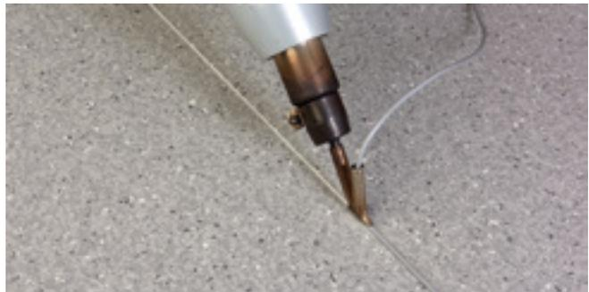
Figure 2 Applying the weld
