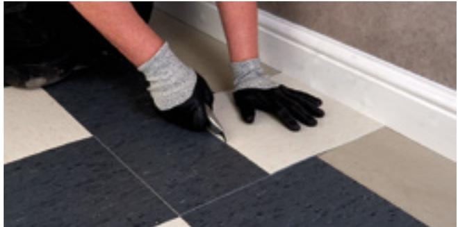
Figure 5 Measuring using an overlapping tile
