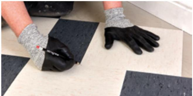
Figure 7 Marking the perimeter tiles (diagonal cut)
