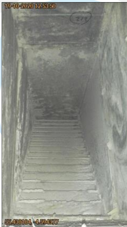
Supply duct before cleaning
