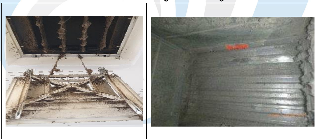
Heavy Contamination on grille and damper.
