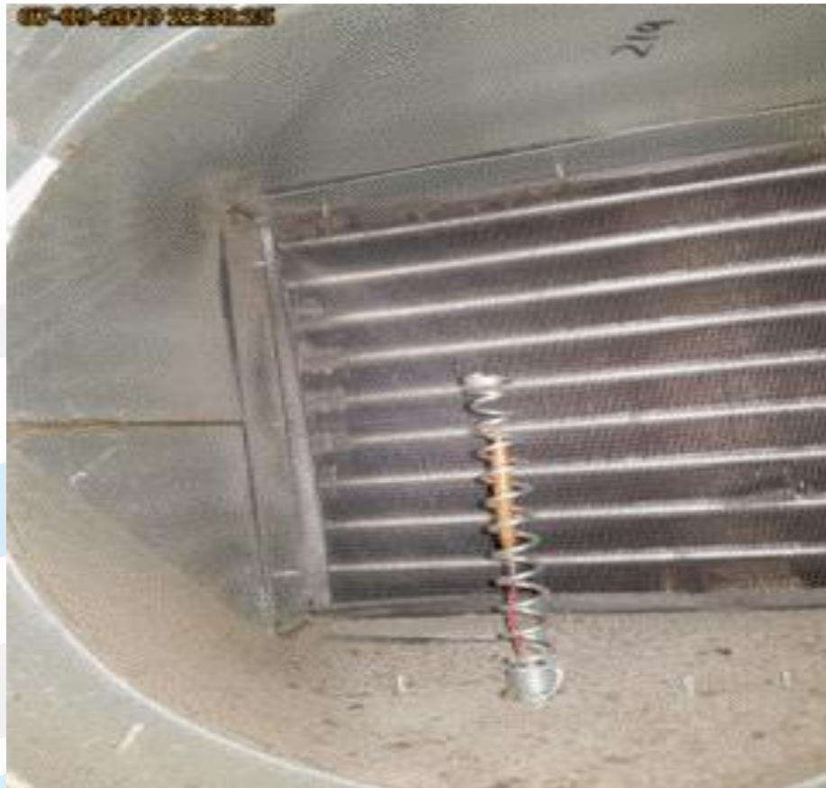
Heavily contaminated and blocked heating coil
