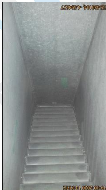
Supply duct after cleaning
