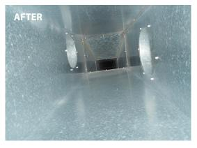
With the use of a variety of extraction devices along with specialised mechanical brushes, air jets and manual cleaning methods, Hygiene Contracts can remove all types of contamination where microbiological contamination is an identified issue and we will disinfect where necessary.
