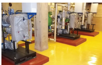
Figures 4 and 5: Good ALARP practice for healthcare? – respectively plate heat exchangers for hot water with no storage, and flow-through type expansion vessels.
