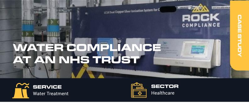
When a large NHS Trust in the South West first wanted to install an additional system to support its existing water compliance control scheme, Rock Compliance recommended Copper and Silver Ionisation. Seven years later, this is now the method used successfully across the site.
