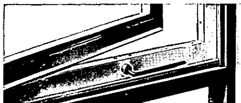
The window and key in the locked and unlocked positions.
