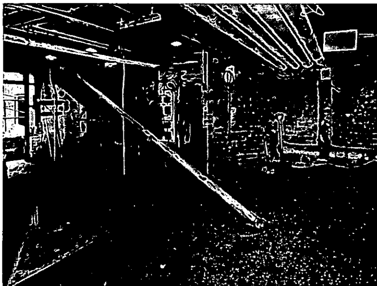
The Mayrath Conveyor to simplify and speed up the loading of the boilers.
