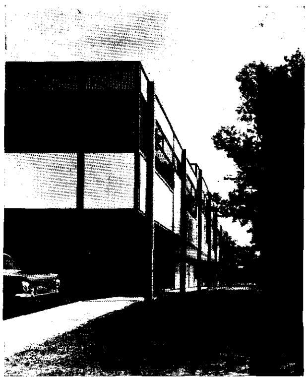
A view of the fully exposed steelwork and vitrolite cladding.
