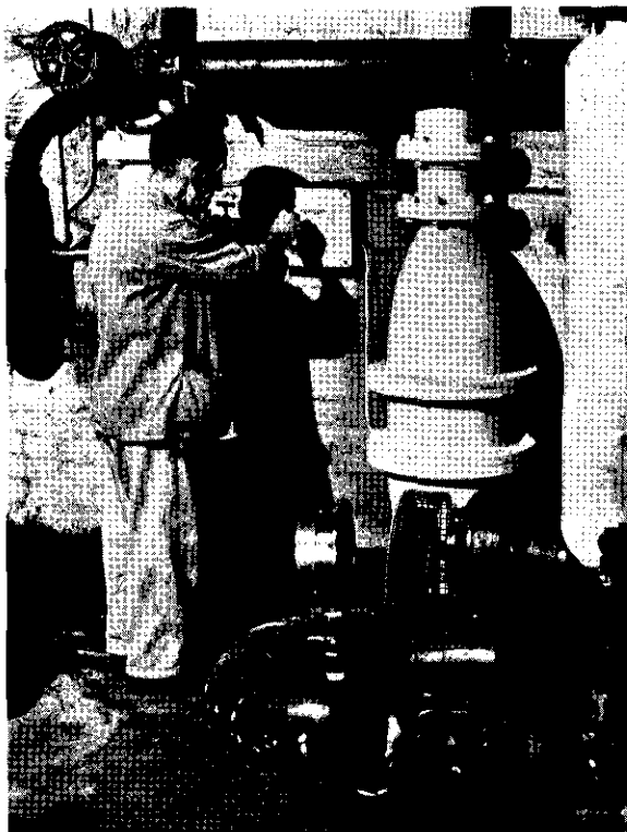
Fig. 1. The only maintenance the Aquastat requires is to check the control box setting. This is a 6in. process unit at Horton Hospital, Epsom with one of the calorifiers showing in the foreground.
