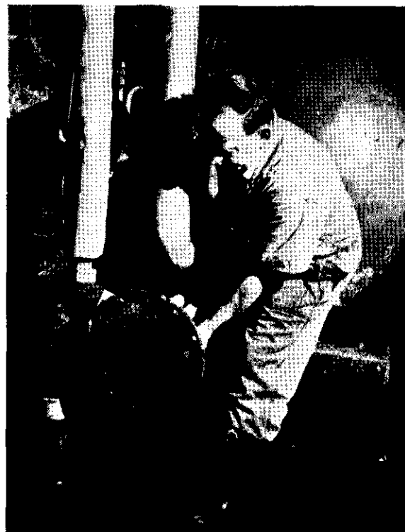
Fig. 2. It took just five minutes to prepare the tubes of this eight-year-old calorifier for the Boiler Inspector after 12 months continuous running with steam-side temperatures at 250".
