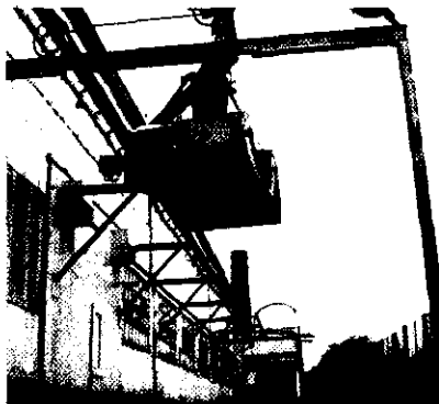
A fully automatic Noiroi (Charrold) handling installation moves coal from storage point to boiler feed hoppers.
