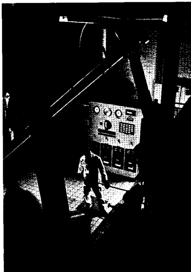
Above: The Control Panel from an unusual angle. This incorporates an audible alarm and visible indicator system for fault finding use should these occur.
