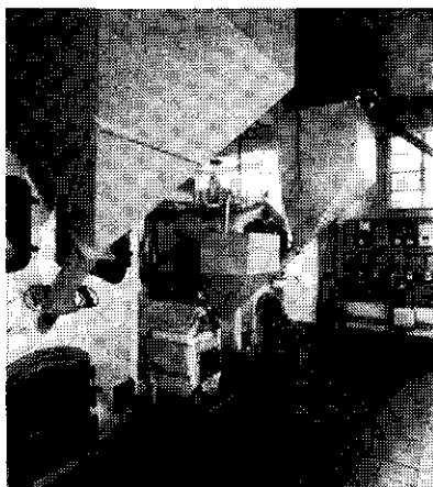
Gravity Feed. A fuel hopper automatically feeds fuel to the firebed, where air is forced in to provide almost total combustion. Removal of the small amount of clinker left by this method, and re-filling of the hopper, takes only a few minutes each day. For large installations, automatic hoppers are available.
