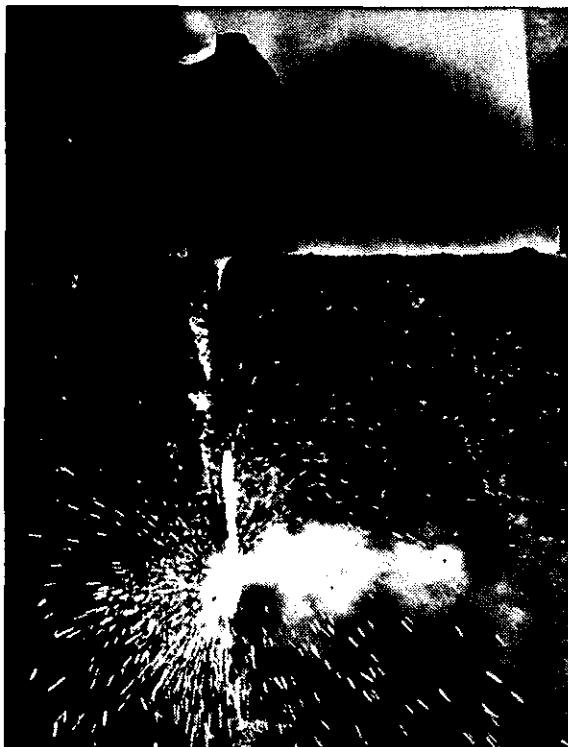
Cutting massive concrete structure at Southampton Docks
