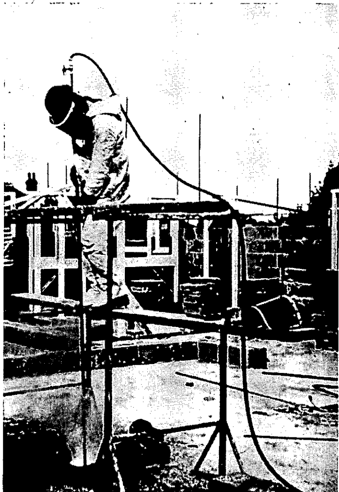
Boring vertical holes with a thermic lance
