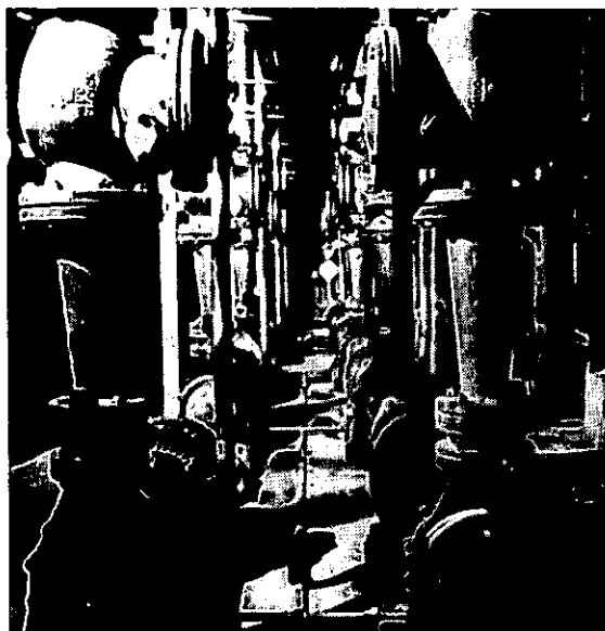
Fig. 2 Eight raw-water pumps laid out in a row between the filters
