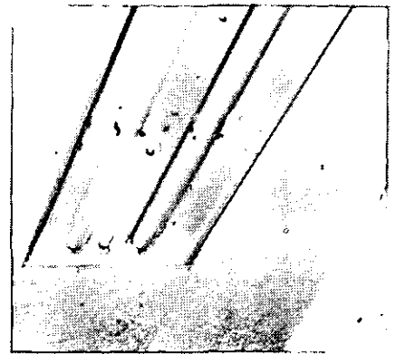
Figure 4b Interior view of a luminaire of the type shown in 4a. The miniature fluorescent tube, operated from a 24V central battery emergency system, can be seen between the mains tubes. (Poselco Ltd. for Modular Support Systems).
