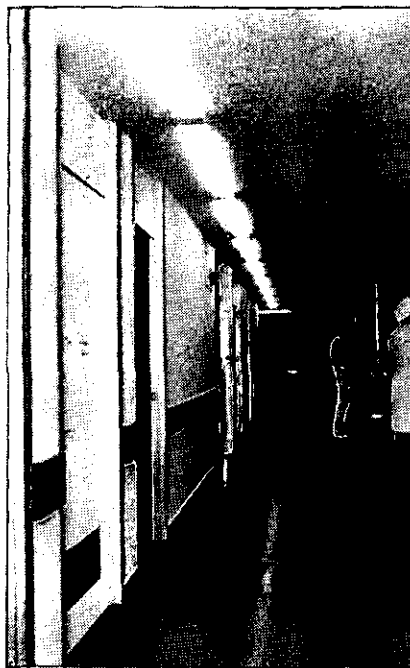
Figure 4a Recessed fluorescent fittings of a design which can incorporate additional lamps for emergency purposes where required.
