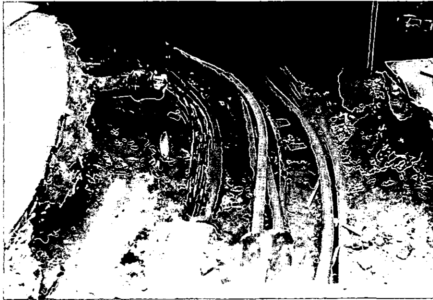
Cable ducts broken back to expose cables.
