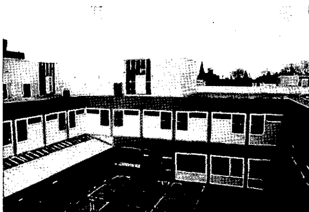
Figure 12. Roof. Guard rails should be provided here to ensure access in such positions.
