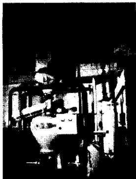
Coal feed and ash removal system. Transmitton's boiler controls.
