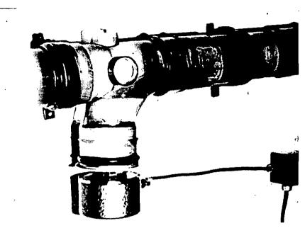
Figure Eight: Drain blockage indicator.
