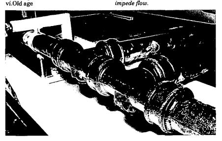
All bends must be of large radius, preferably a combination of two 135° angles, if rough bore pipework is specified.
