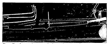
Figure Five: Incorrectly supported polypropylene pipework.
