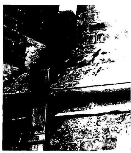
Figure Ten: Defective down pipe set in masonry.
