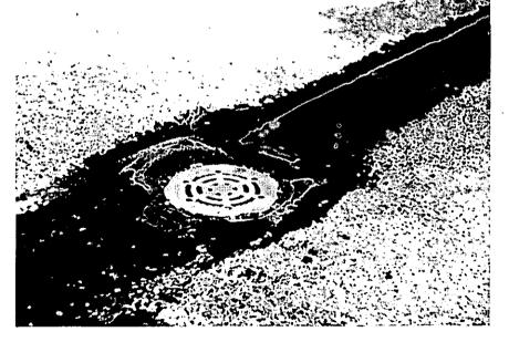
Figure One: Settlement damage to the roof membrane.
