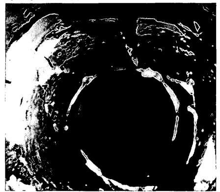
Figure Nine: T. V. identification of broken clay drain.
