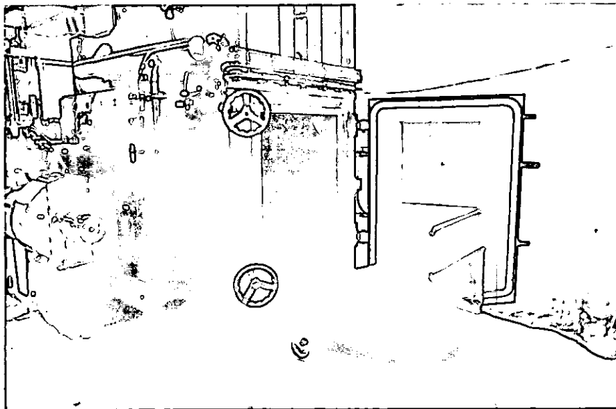
Typical arrangement for manual ash removal
