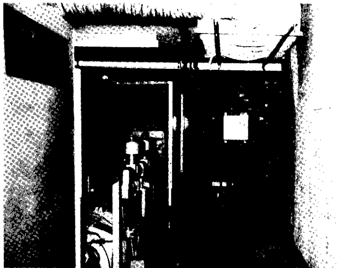
Figure 1 illustrates a typical installation with the wall mounted Cyclic Loading Unit (8) sited as close to the generator as possible.
