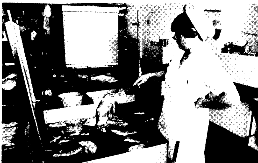
Fish frying takes place in the central cooking area at Maidstone. It is accessible and easily cleaned with plenty of extract ventilation.
