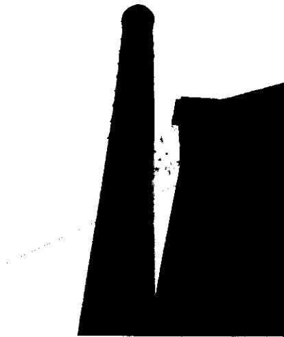
Victorian hospital chimney badly leaning and hooped, just prior to demolition.
